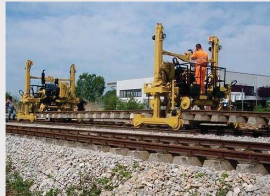
Switch replacing
